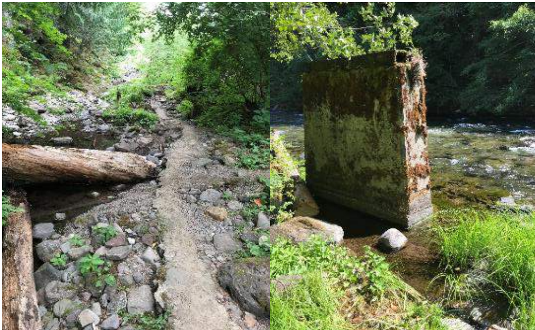
Figure 5. Concrete remnants within Clackamas River channel
