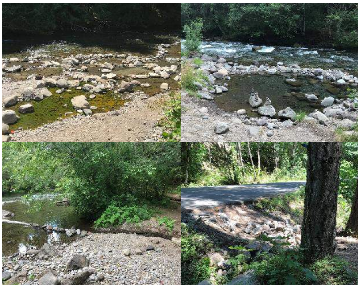
Figure 14. Photo Group C: Improvised River and Roadway Alterations
