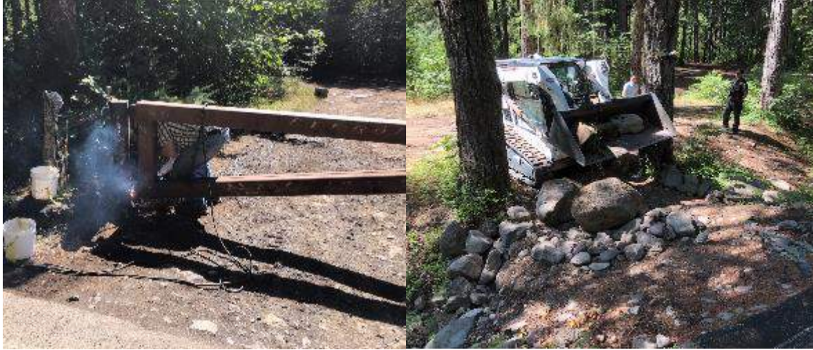
Figure 4. Main gate reinstallation and access point barrier along FSR 46
